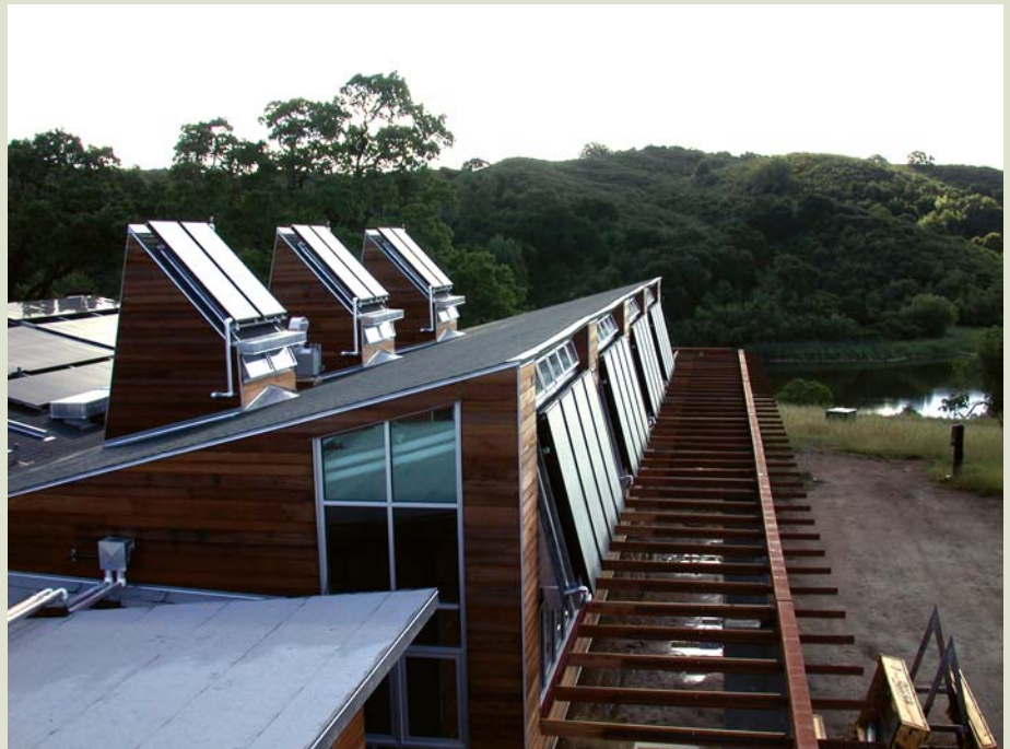
This 22-kilowatt photovoltaic system, consisting of 275 80-watt BP Solar TF-80B thin-film modules, provides most of the power for the 9800-square-foot research and teaching facility.
